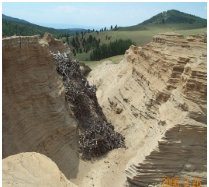
Example of the damage done to Four Mile Creek near Victor and Cripple Creek.
